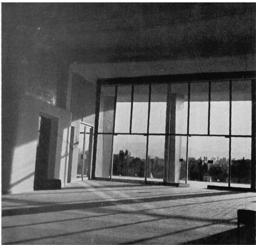
Forefront Building Public's Entrance
